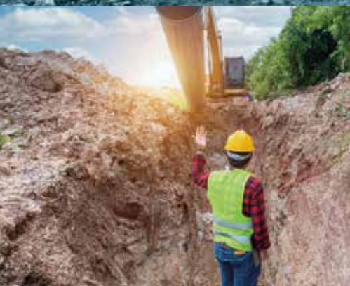
Mining and road construction
